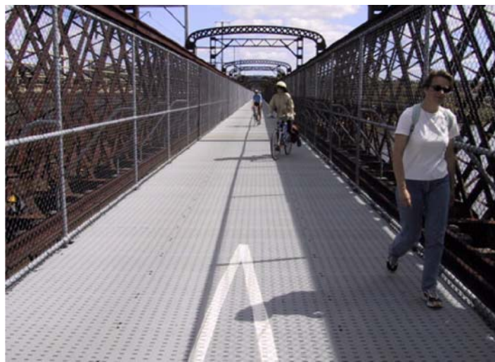
Figure 5: Recent infrastructure for bicycles - John Whitton Bridge, Meadowbank, Sydney, which is part of the Concord to Eastwood Rail Trail
