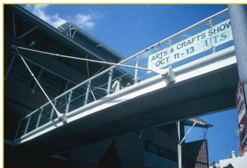
Figure 10: Pedestrian Bridge: Member in tension and bending
