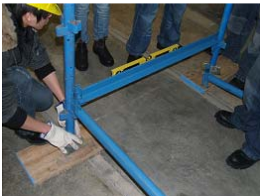
Figure 1: Adjusting vertical screws to ensure ledger is horizontal
