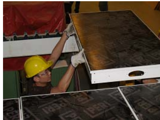
Figure 6: Placing the deck
