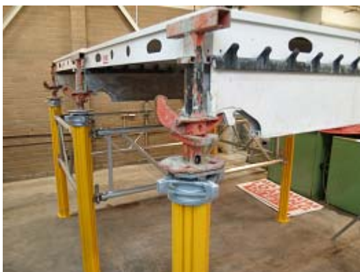
Figure 7: Formwork complete. A drophead is in the foreground ready to be released
