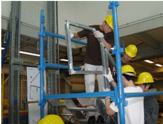
Figure 3: The upper handrail is installed from a lower level protected by the lower handrail
