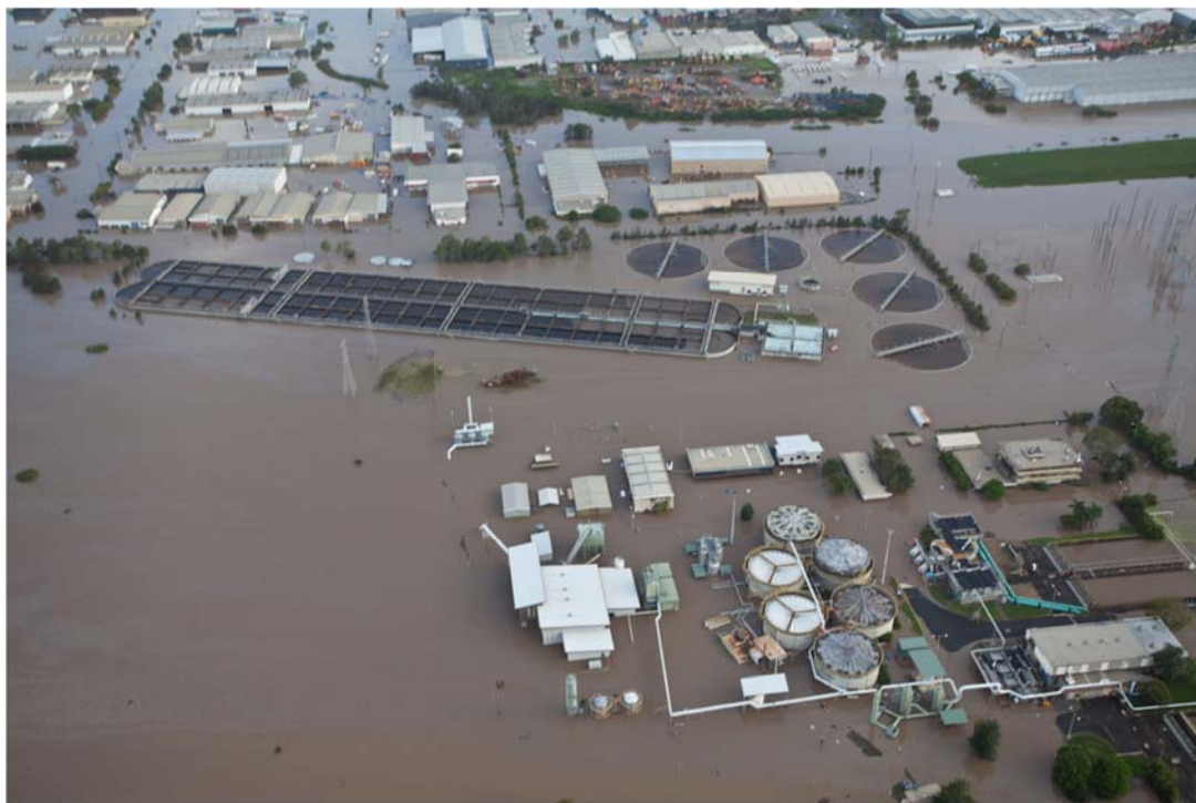
Figure 1: Oxley WWTP used as an example of uncertainty management issues (2010 flood event, photo by Aleks Atrens, copyright preserved, and photo used with permission).
