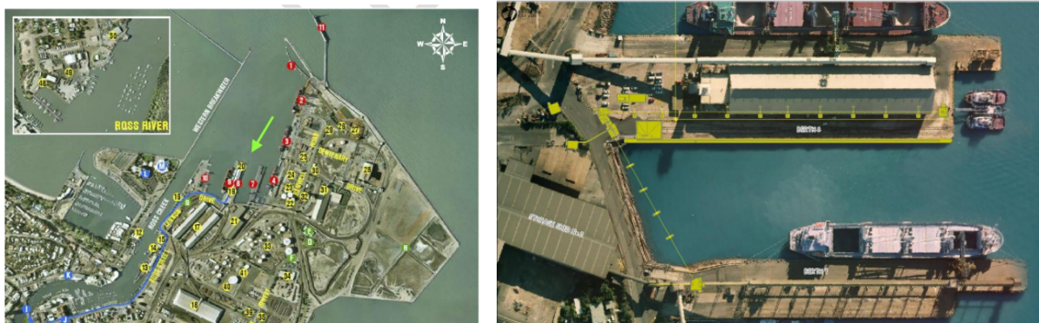
Figure 1(a) Port of Townsville showing location of Berth 8 (b) Details of proposed new infrastructure at Birth 8
