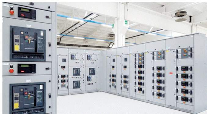
Figure 5: Switchgear Panels in the Substation
