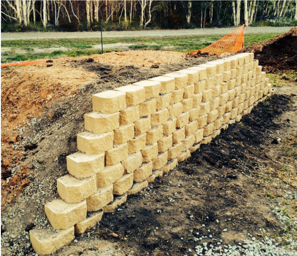
Figure 3: Completed earth-retaining structure, approximately 1 m high.
