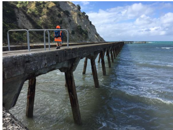
Figure 3: Deteriorated condition of the Tokomaru Bay Wharf
