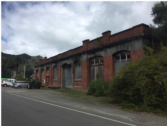
Figure 2: Tokomaru Bay Shipping Company heritage building, another focal point for the project
